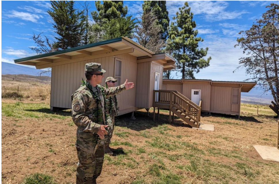
Chief Guy Travis and Captain Esteban Acevedo detail cabin updates to distinguished visitors on a tour of the newly-repaired Camp Kilohana on Hawai'i Island
